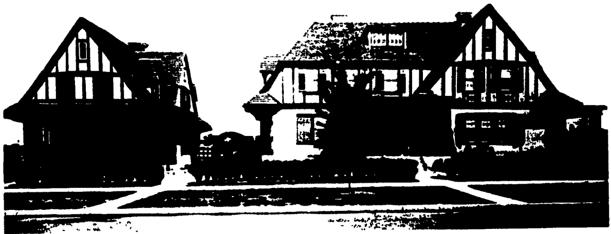
Fig.2.5. Typical Gothic-Tudor Styled Houses at Forest Hills Gardens (Stilgoe, Borderland )
