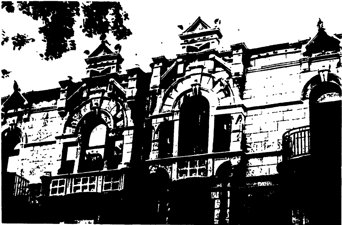
Fig.3.2. Greystone Terrace Houses on Dorchester Boulevard (Renovation in Westmount )
