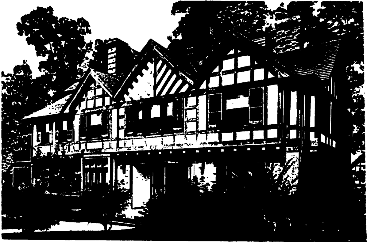
Fig.2.3. A 'Tudor' Styled House at Roland Park (Howland and Spencer, The Architecture of Baltimore plate)
