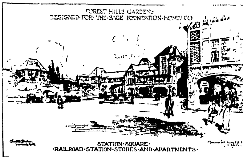
Fig.2.4. Station Square at Forest Hills Gardens ("Forest Hills Gardens," The American City )
