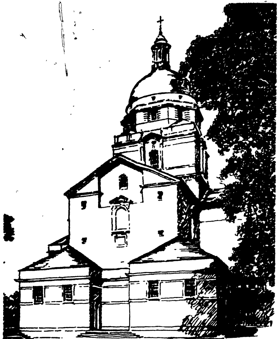
Fig 4.78 The Cathedral Church of the Redemption
