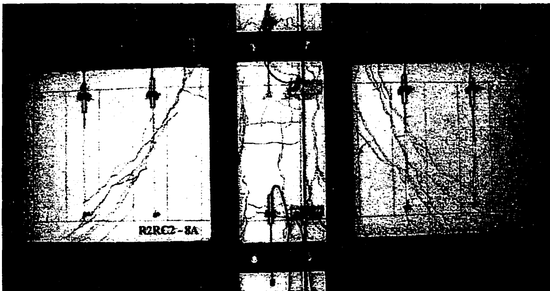
Fig. 5.18: Distress in Spandrel beam of Specimen RS2
