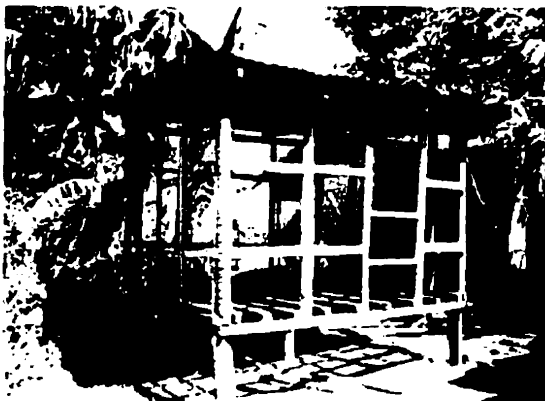
Fig. 4.2L Example of timber framing Source: Photo by author.
