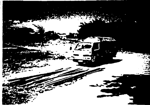
Fig.4.3s Trucks unload the materials at the entrance to the community. Source: Photo by author.
