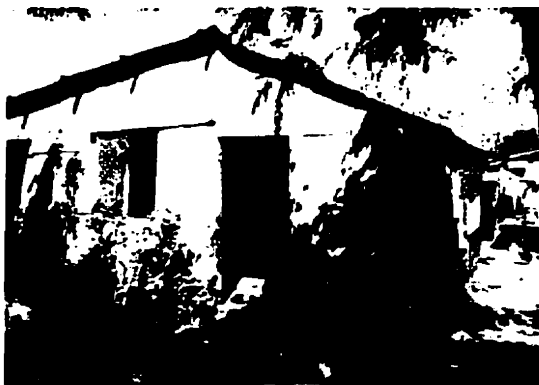
Fig. A.3 Exterior view of the house. Source: By author.
