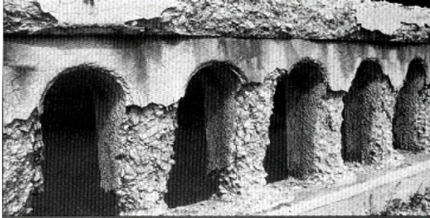
Figure 1: Typical example of concrete deteriorated from freeze-thaw actions (non-air entrained concrete railing)
