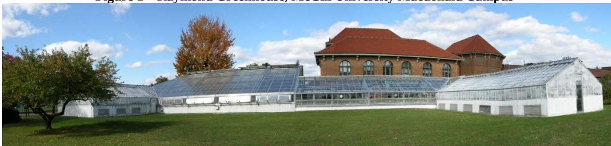
Figure 1 – Raymond Greenhouse, McGill University Macdonald Campus
