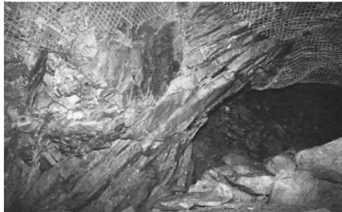
Figure 2-2. Spalling driven by stress raisers in the corner of an excavation (Moss and Kaiser, 2021).
