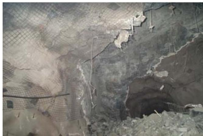
Figure 2-3. An example of shearing along structure generating seismic damage (Heal et al., 2006).
