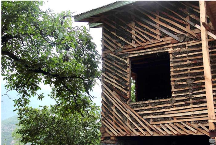
Figure 2-44 Wood structure of a Zogali wall. Source: personal archive of Mr. Ali-Esmaeeli
