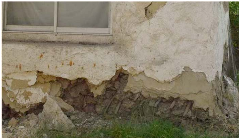
Figure 2-45 Water has washed the mud of a Zogali wall Photo by author
