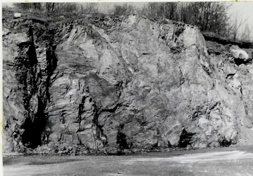
Figure 10. Typical view of Face # 7 Wall is 20 ft. high.
