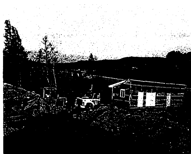
Figure 2.6 Transporting modular units (Scanada Consultants, 1996)
