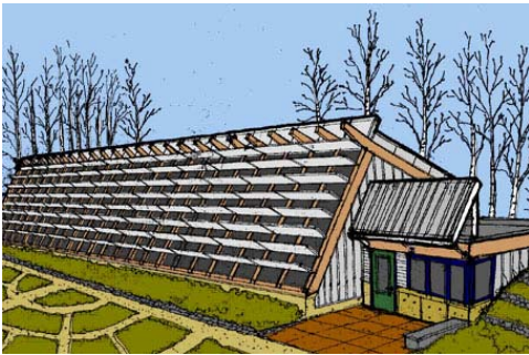
Solar aquatic wastewater treatment facility
