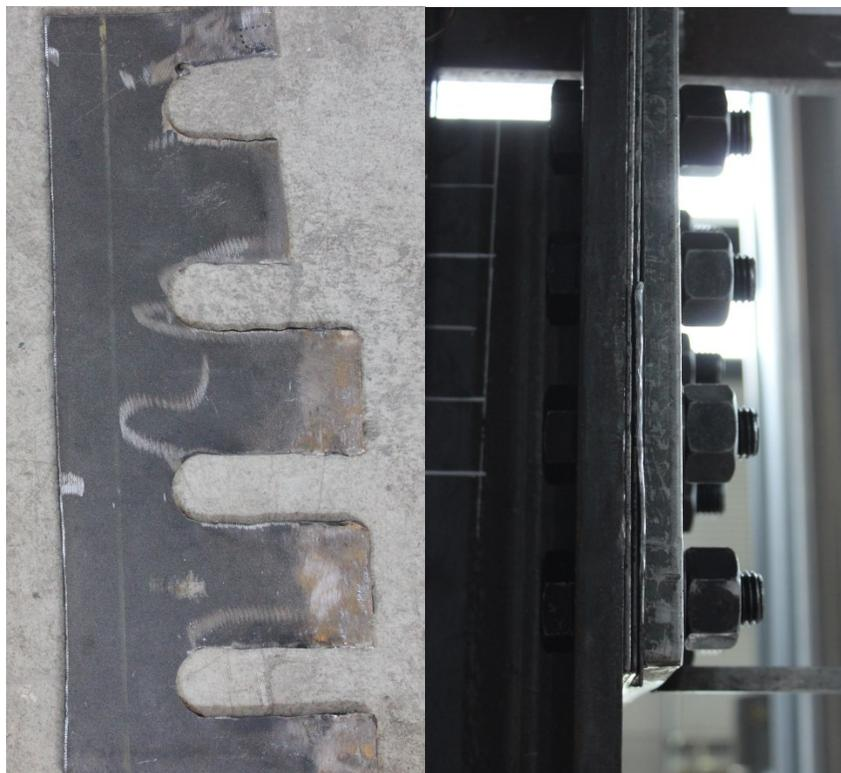
*Figure 4-6 Modified shim plates (left) and shim plates in assembled connection (right)*
