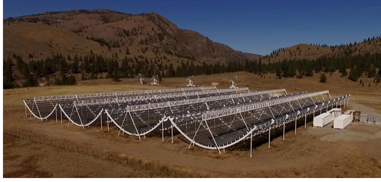
Figure 2.1: Photo of CHIME taken from CHIME/FRB Collaboration (2018) showing the four cylindrical reflectors and the shipping containers on the right which house the X-engine and the FRB search backend.
