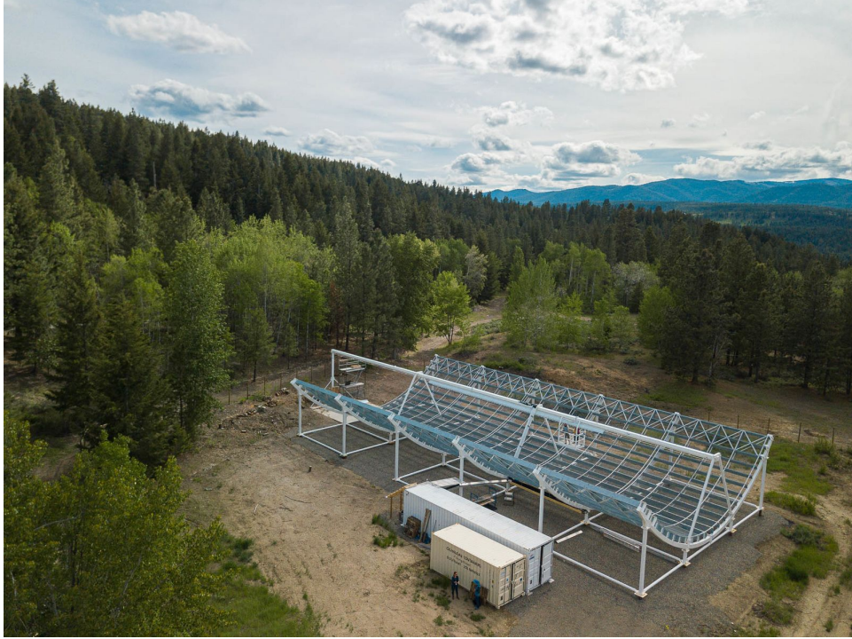
Figure 4.1: Aerial view of KKO. The receiver hut on the side houses the F-X engine. The trolley attached on the focal line allows easy access to the feeds for assembly and maintenance.
