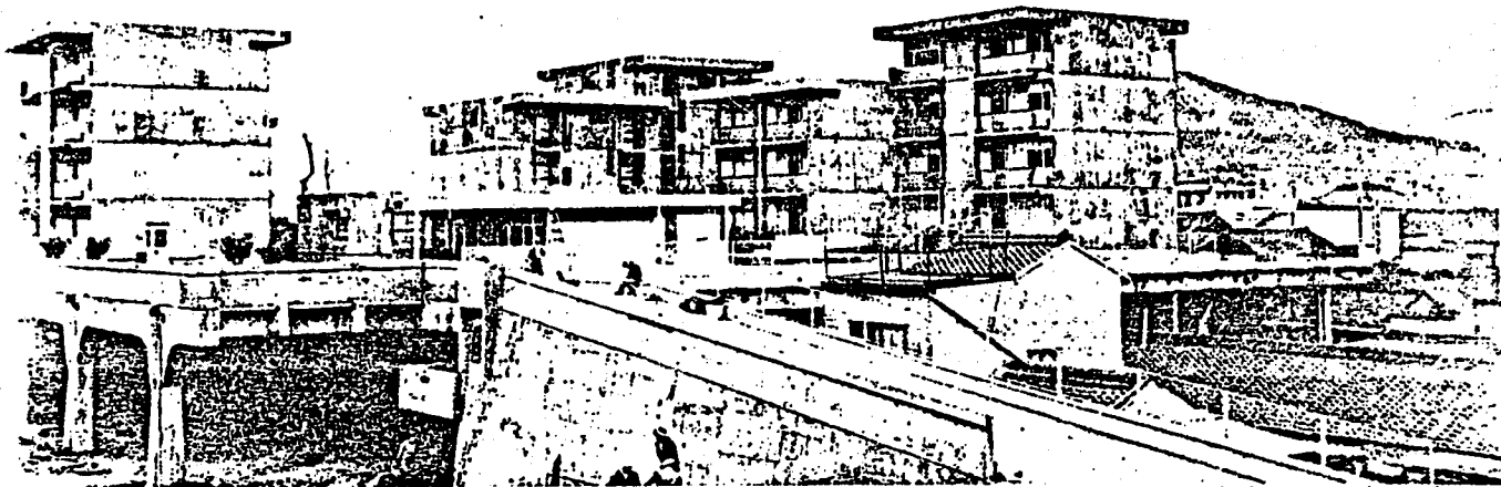
st-chloride panel from the of the apartments.
