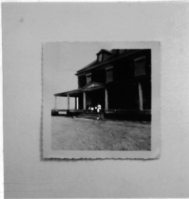
Photo 25: Idlewyld with blocked-up windows
