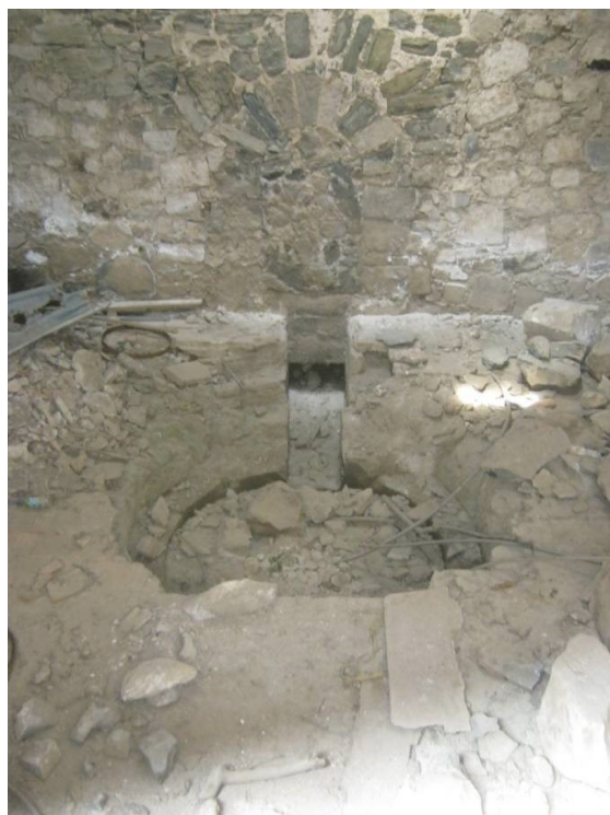
Figure 4-16. Tentative location for a capellina , showing the channel for cooling water. This picture was taken in March 2013. Further excavation around this location has been carried out by November 2014.
