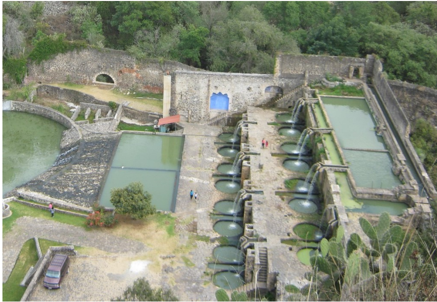
Figure 4-9. View of the sixteen circular vats of the arrastres . The remains of two molino tracks are hidden by the cactus leaves on the lower right-hand corner.
