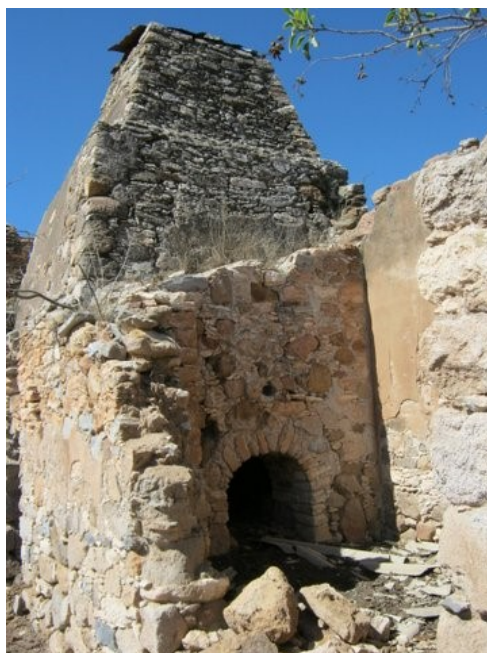
Figure 2-3. Exterior of smelting furnace at the ruins of the Hacienda Santa María in Monte Caldera. The arched port would have been used to feed ore or fuel to the furnace.
