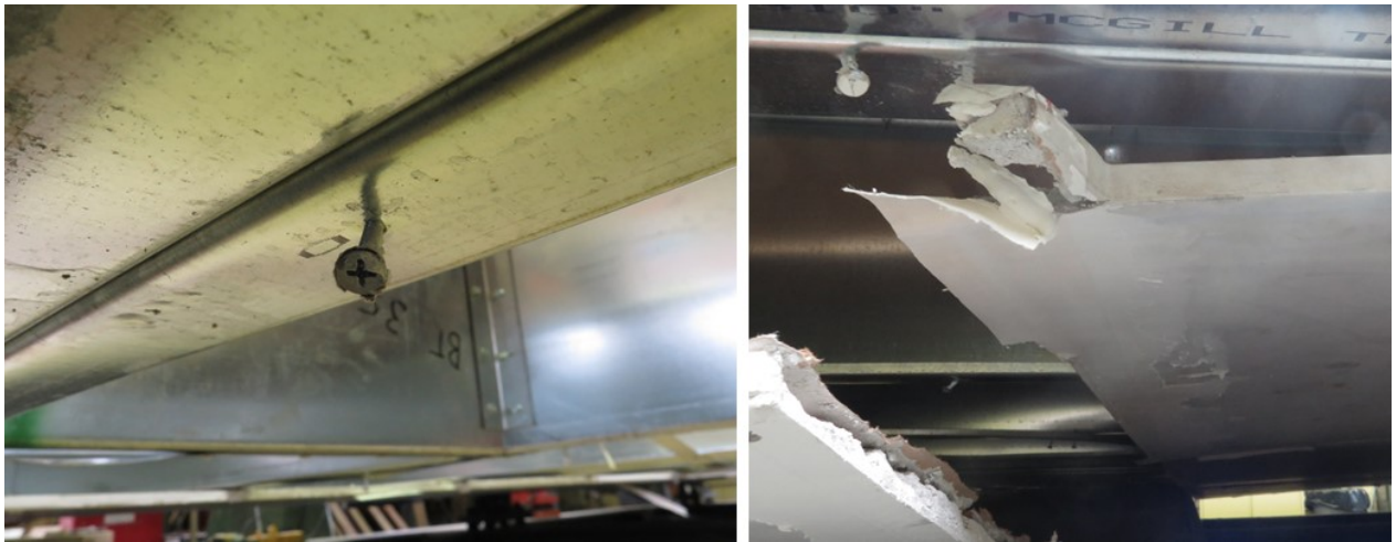
Figure 3.27: (Left) Tilted Gypsum Fastener, Gypsum Panel Had Fallen (Right) Tear out of Gypsum Fastener at Corner Location
