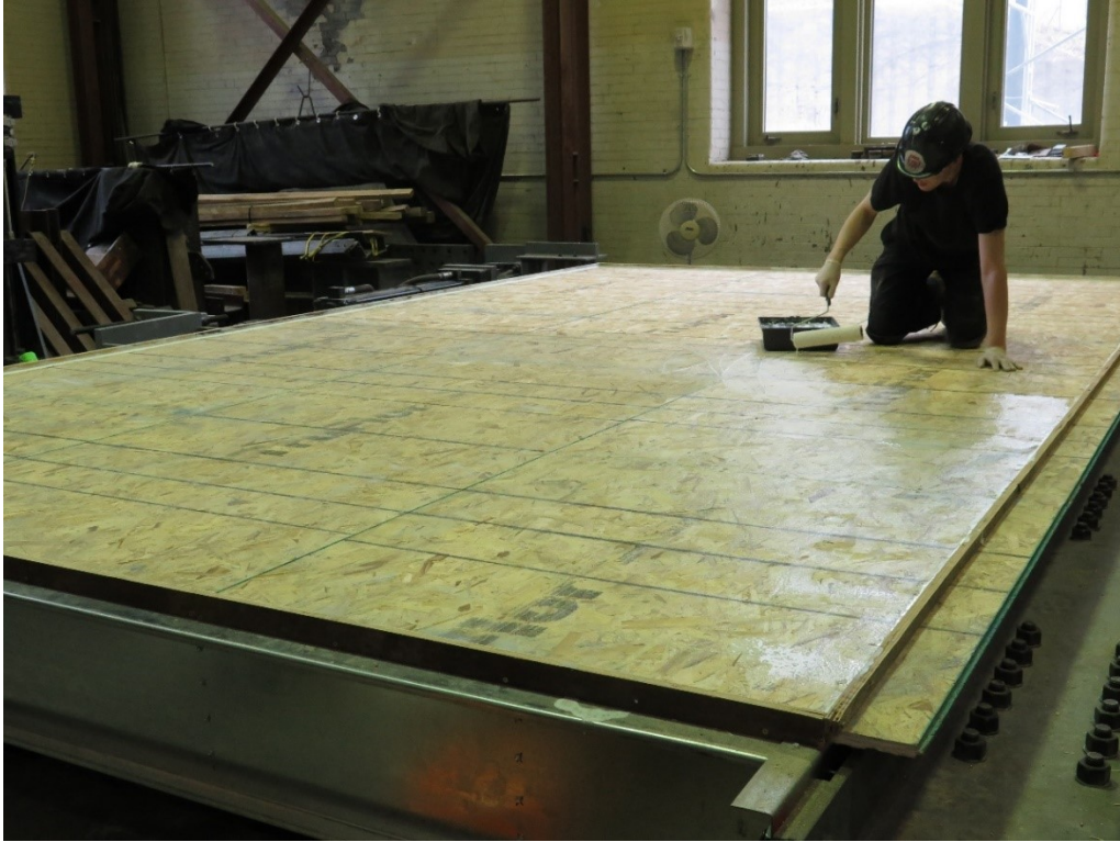
Figure 2.22: Application of First Coat of Floor Primer to OSB Sheathing
