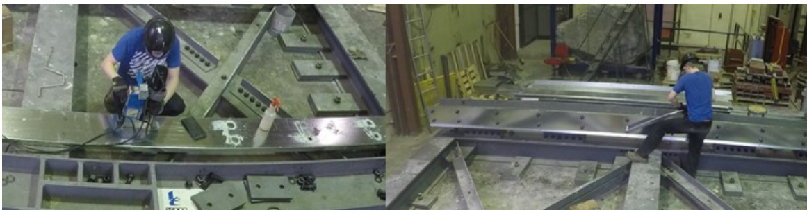
Figure 2.12: (Left) Drilling Holes with Magnetic Drill (Right) Snug-Tightening Rim Joist to Frame Using Elongated Ratchet
