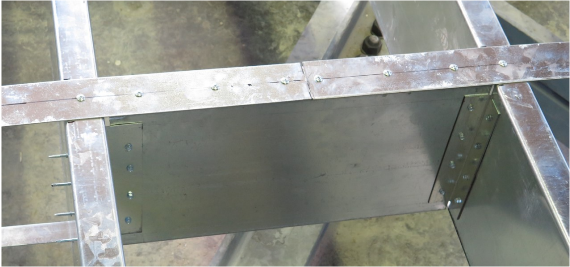
Figure 2.19: Strap Splice Interface at Mid-Span of Blocking Member
