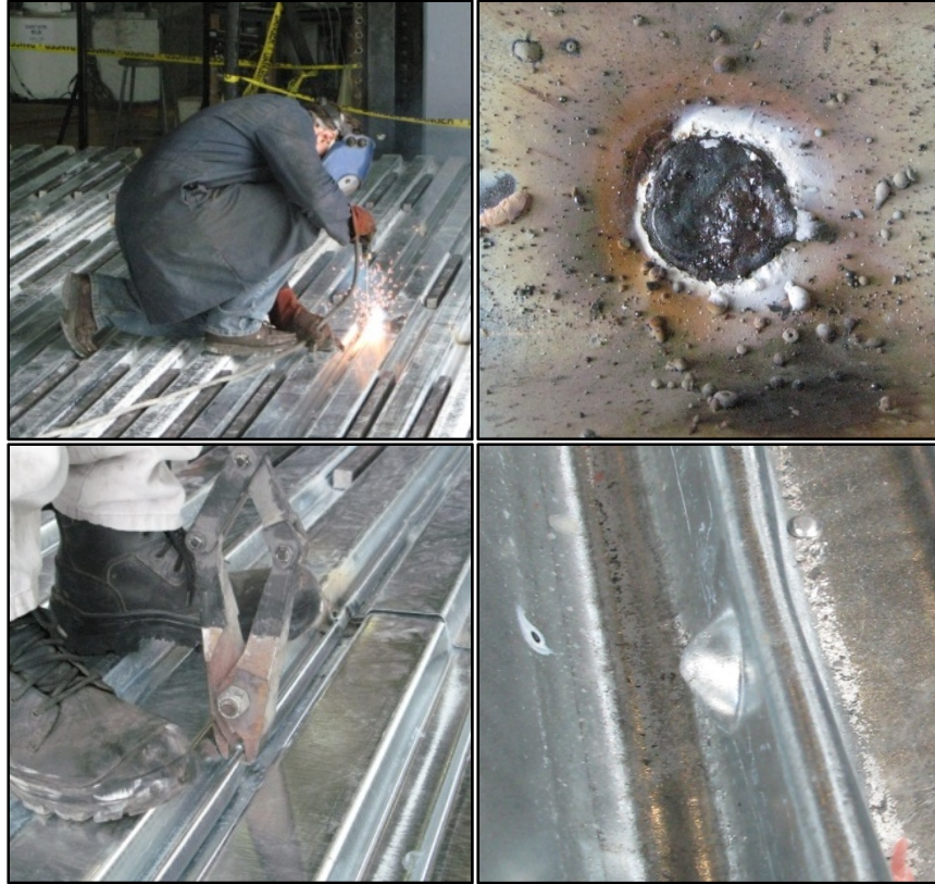
Figure 2.12 – Non-mechanical sidelap fasteners during and after installation
