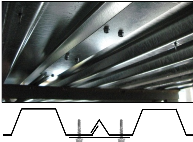
Figure 2.16 – Screwed steel strip repair of button-punched connections
