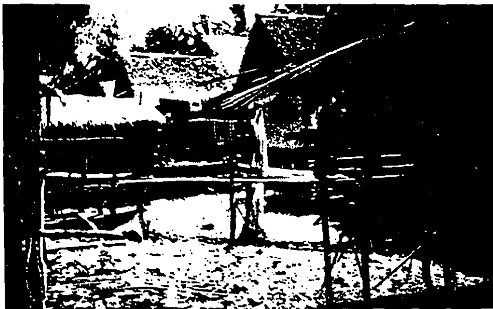
Figure 5.4: Houses located on transition and water zones are supported on stilts with the floor level of the houses at least a meter from the high tide water level.
