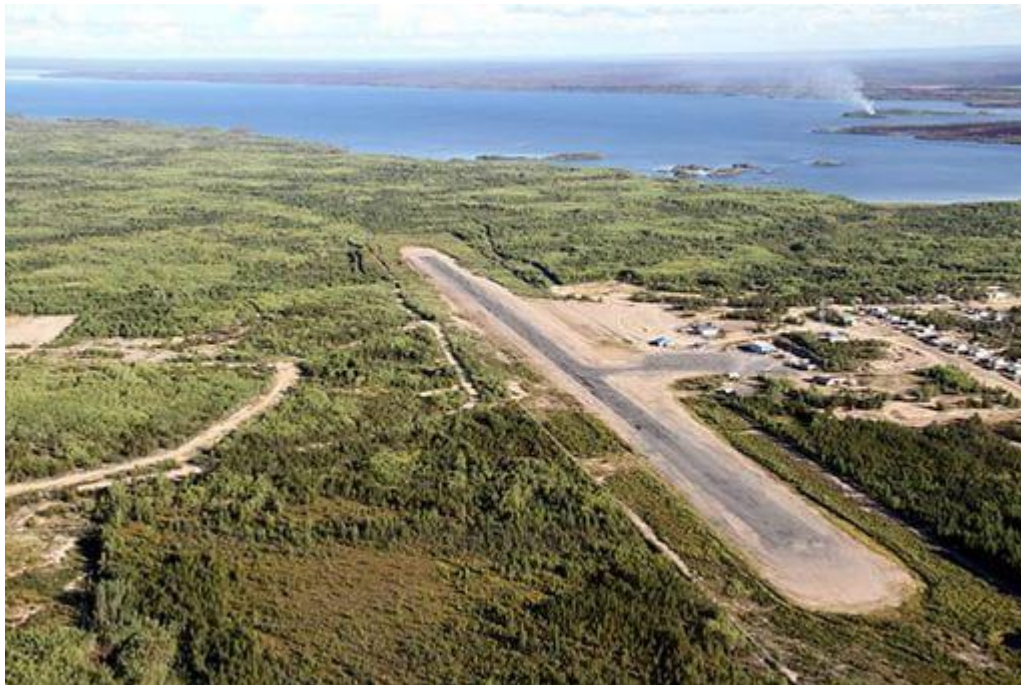
Figure 6—Fond-du-Lac Airport (CZFD)
