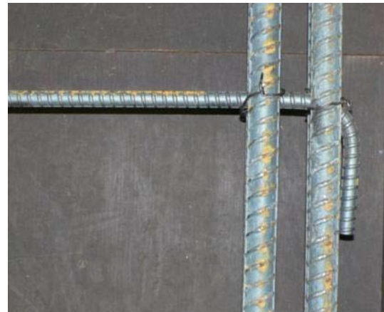
(b) detail of the single-leg transverse reinforcement
