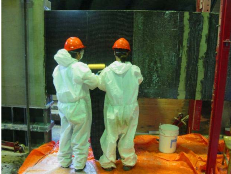
(a) Installing CFRP wrap
