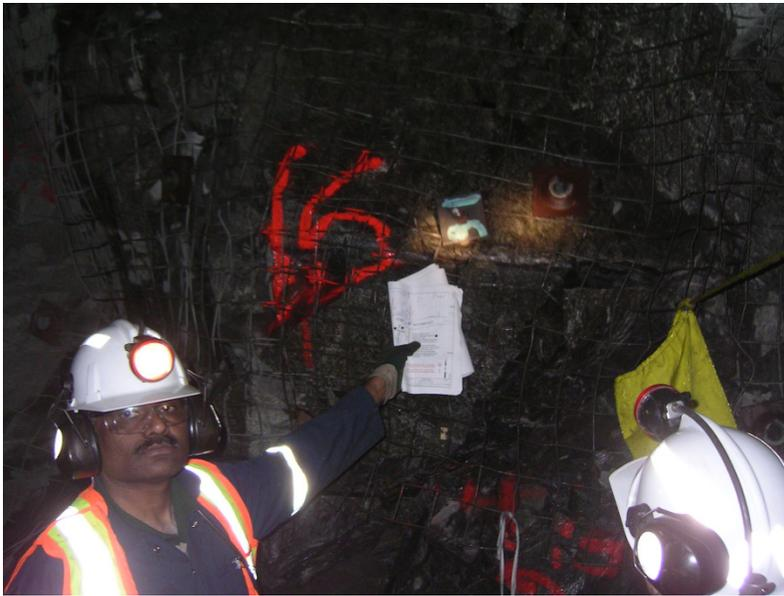
Figure A2-5 Installation of U-Cell in drift wall
