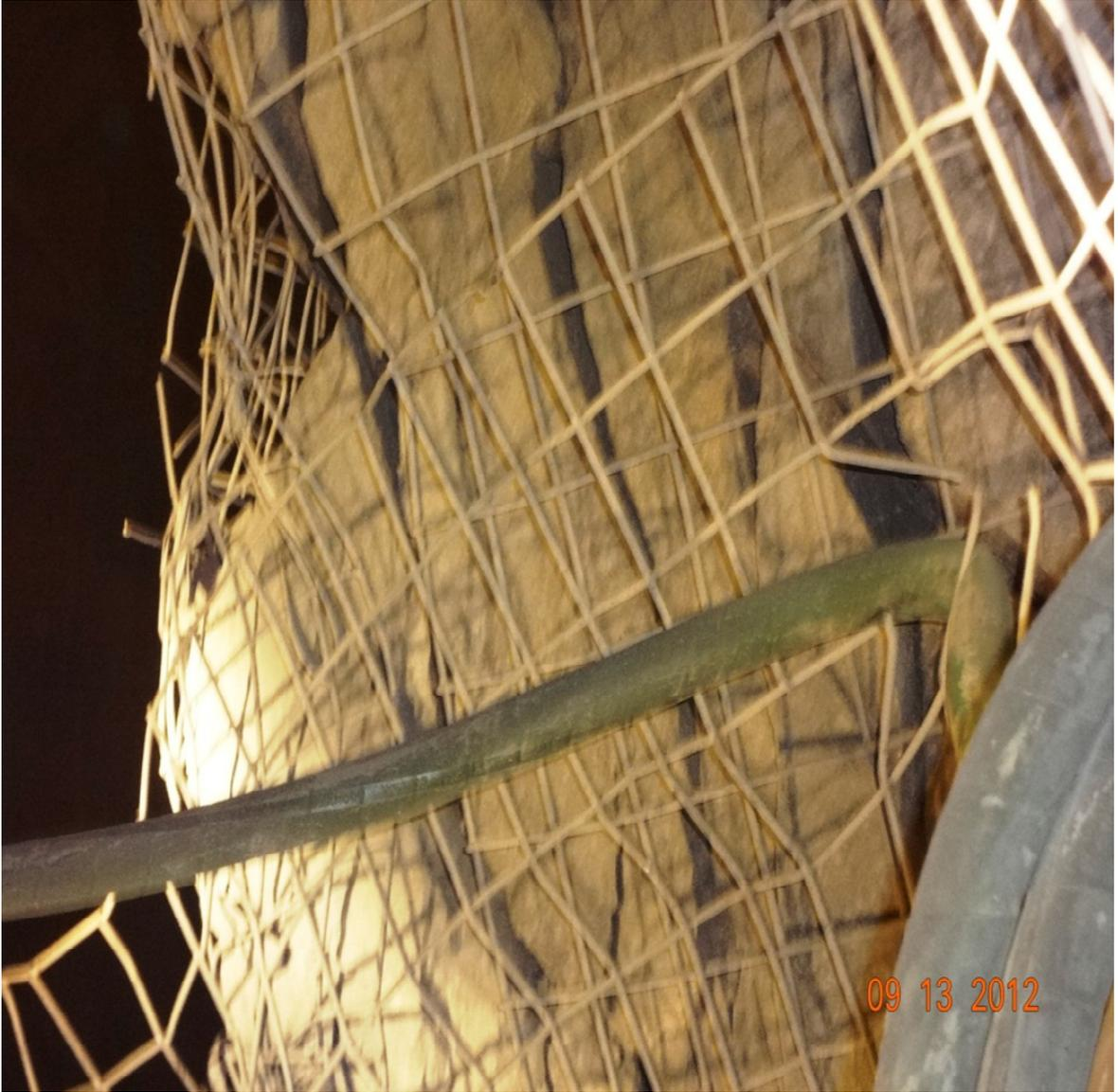
a) Surface rock damage at MPBX location
