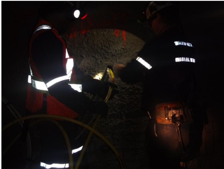
Figure A2-4 Installation of MPBX in drift wall
