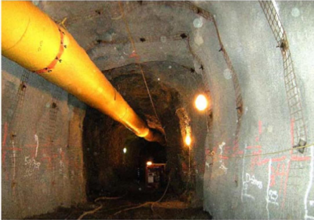
Figure 7-2 Enhanced supports installed in burst prone area (Yao et al, 2009)
