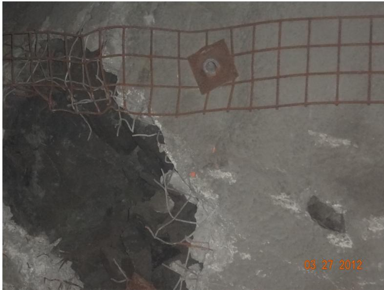
Figure A2-3 Drift wall condition before and after miner rockburst
