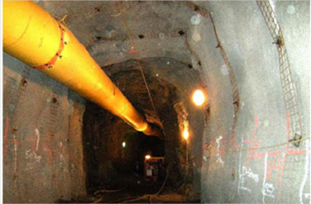
Figure 2-8 Enhanced supports installed in burst prone areas (Yao et al. 2009)
