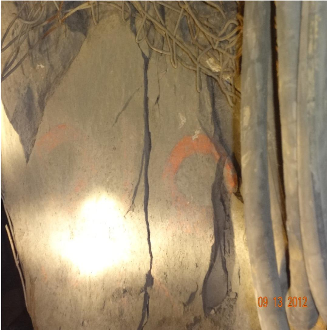
b) Rock fracture near the MPBX location
