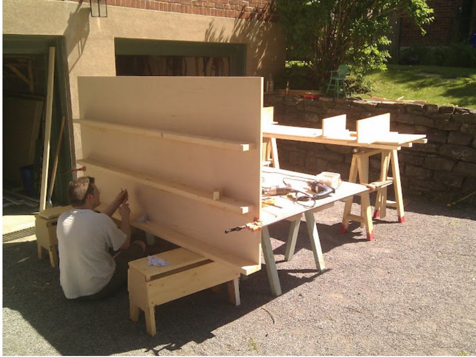
Figure 3.3: The bouldering wall in construction.
