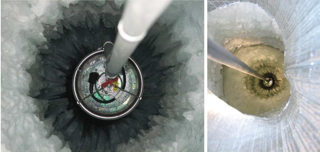
Figure 3–3: The deployment of a string of PMTs in the ice [17]. Each of the 86 holes were dug using a hot water drill. The average time required for drilling and reaming a 2500-meter hole was 30 hours. The holes had a diameter of approximately 60 cm and a lifetime of 24 hours before closure from refreezing. The insertion of the string of PMTs under the ice then required approximately 11 hours.
