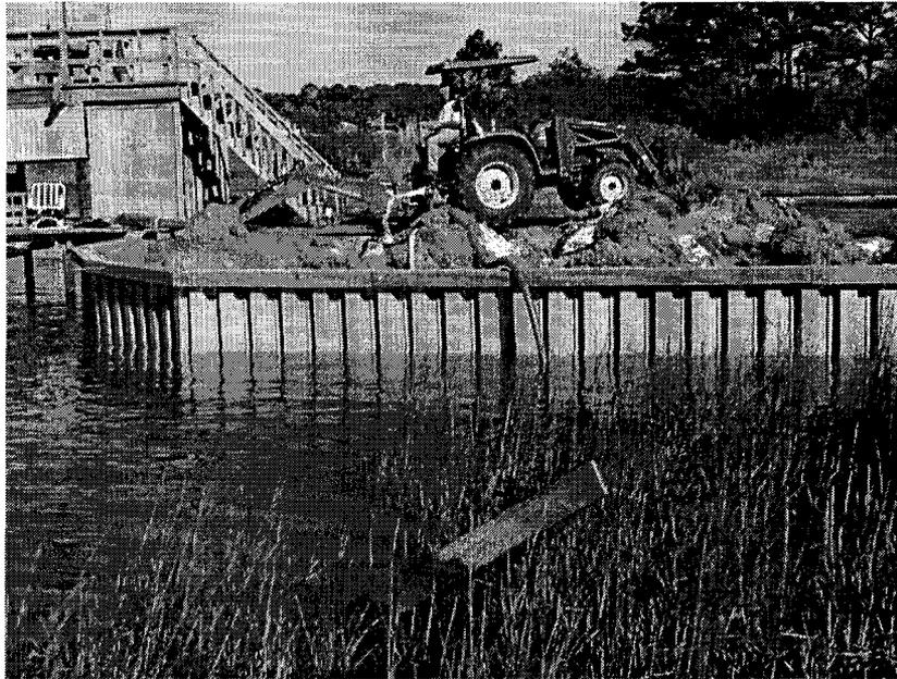
**Figure 1.4:** Backfill material added behind the sheet pile wall.
