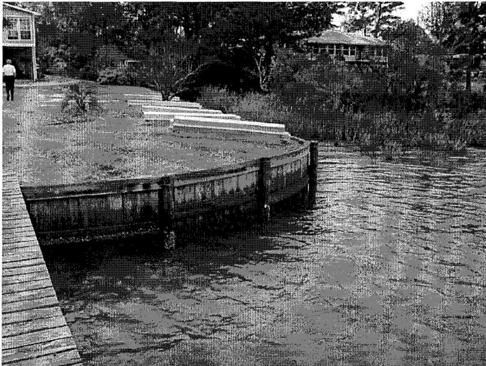
**Figure 1.1:** Replacement of existing decaying timber pile wall
