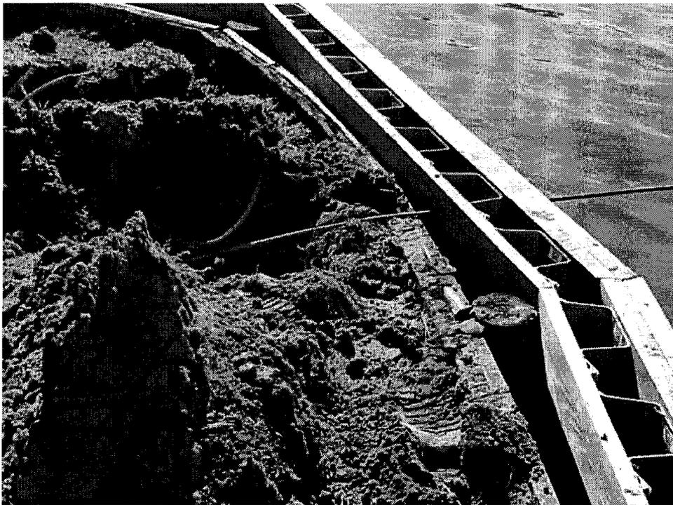
**Figure 1.3:** Anchor system positioned at the top of the sheet pile wall
