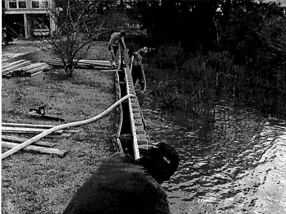
**Figure 1.2:** Insertion of composite sheet piles, (man height not exceeded)
