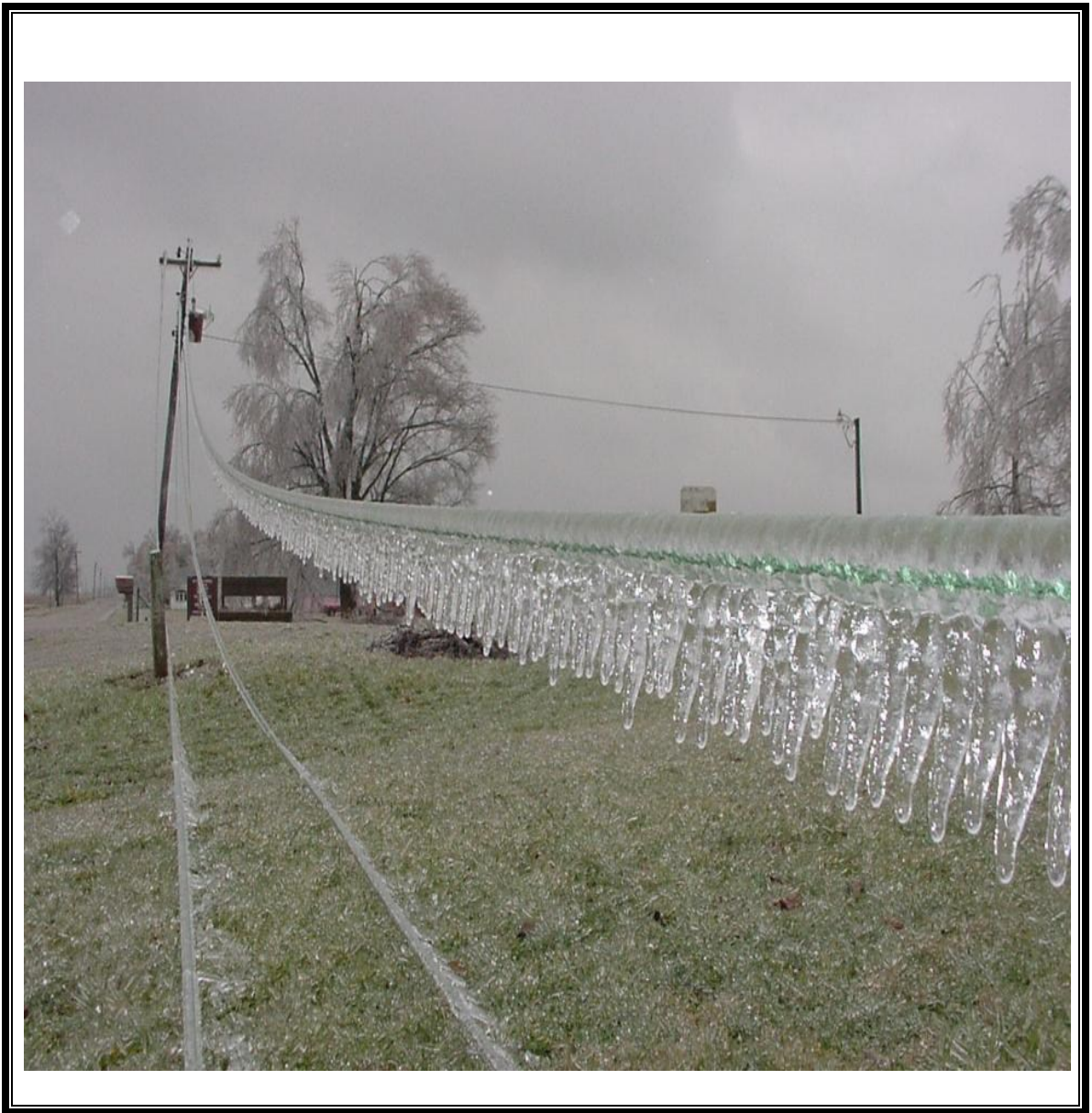
Figure 1.1 Glaze icing on overhead distribution line (source: Brownstown Electrical Supply Co., Inc.)
