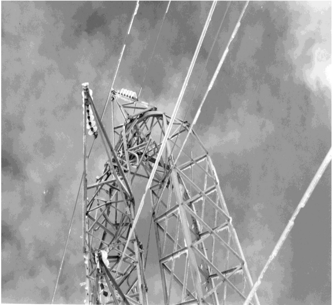
Figure B.2 Close-up view of damage at suspension tower#3 (Source: Hydro-Québec)
