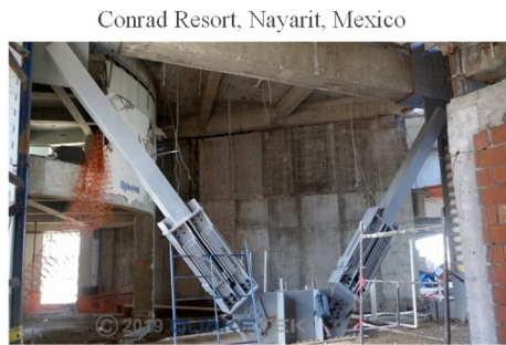
Figure 2-9 Examples of buildings with installation of friction dampers (Quaketek, 2023)
