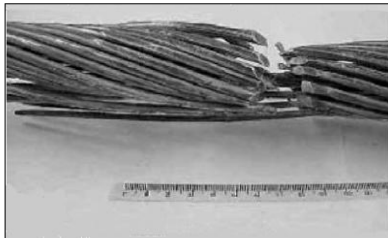
Figure 2.18 General view of fretting fatigue rupture of a ACSR conductor (Azevedo and Cescon, 2002)
