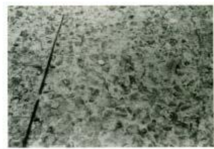
Severe scaling
