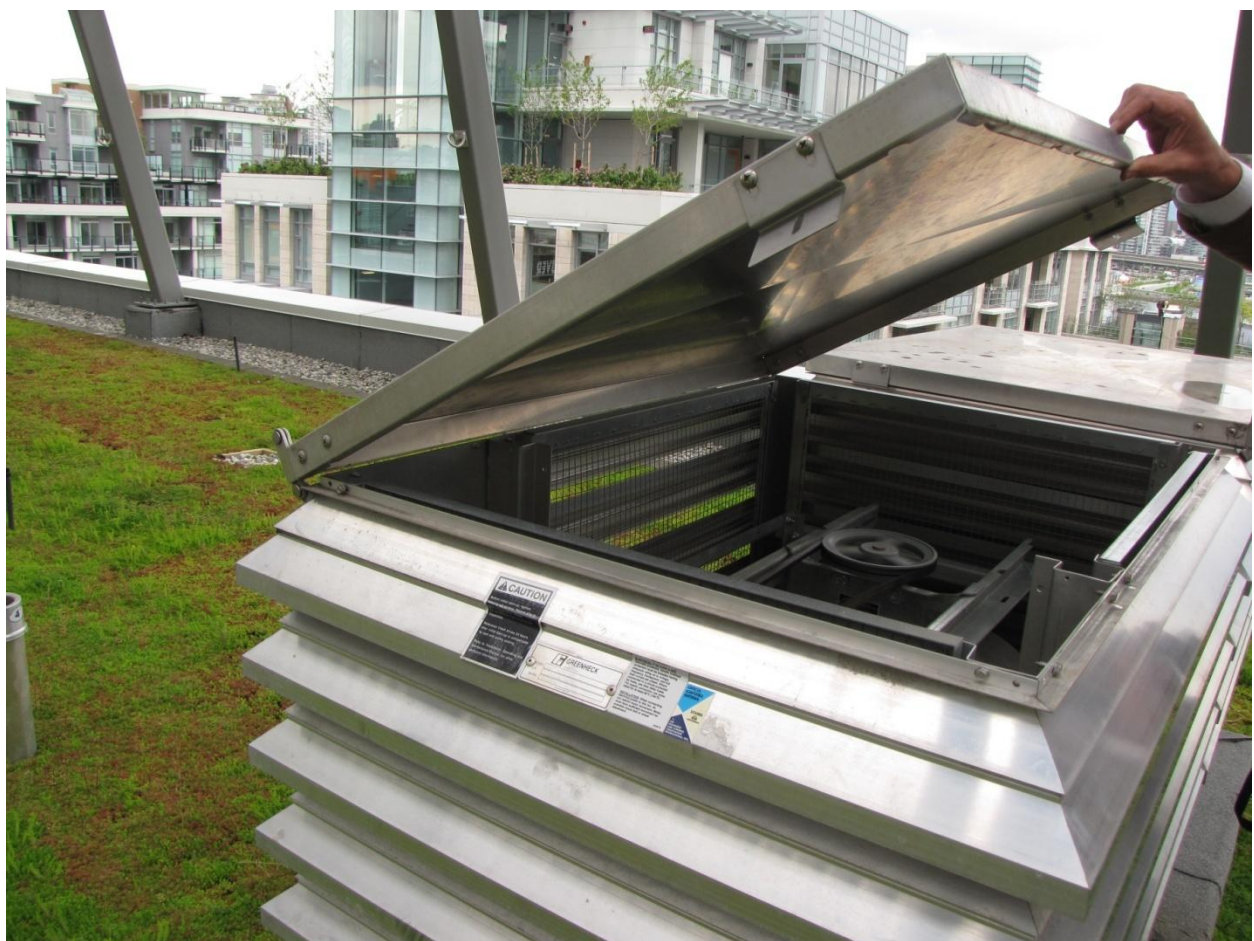
Figure 3-44. Passive Air Shaft on the Roof
