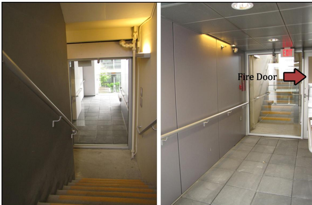
Figure 3-29. The Fire Door Separates the Staircase and the Lobby
