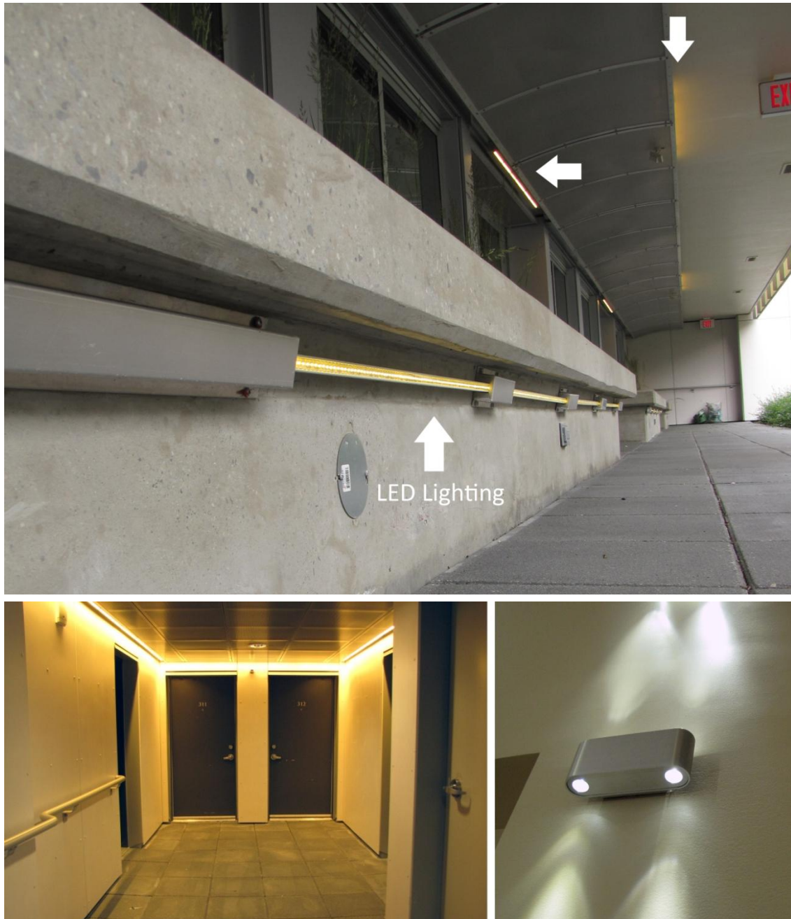
Figure 3-45. LED Lighting in the Indoor and Outdoor Areas On the top: LED lighting in open corridors – At the bottom: LED lighting in the lobbies
