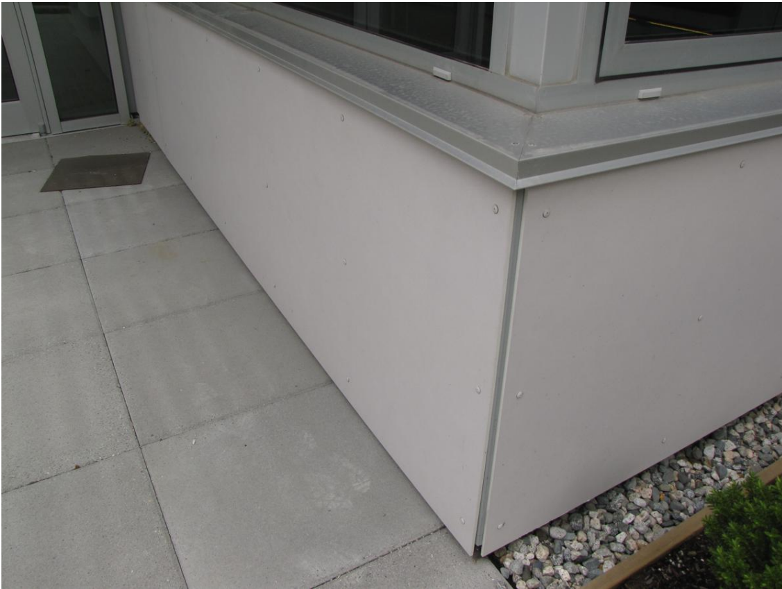
3-48. Cement Boards - Cladding Material
