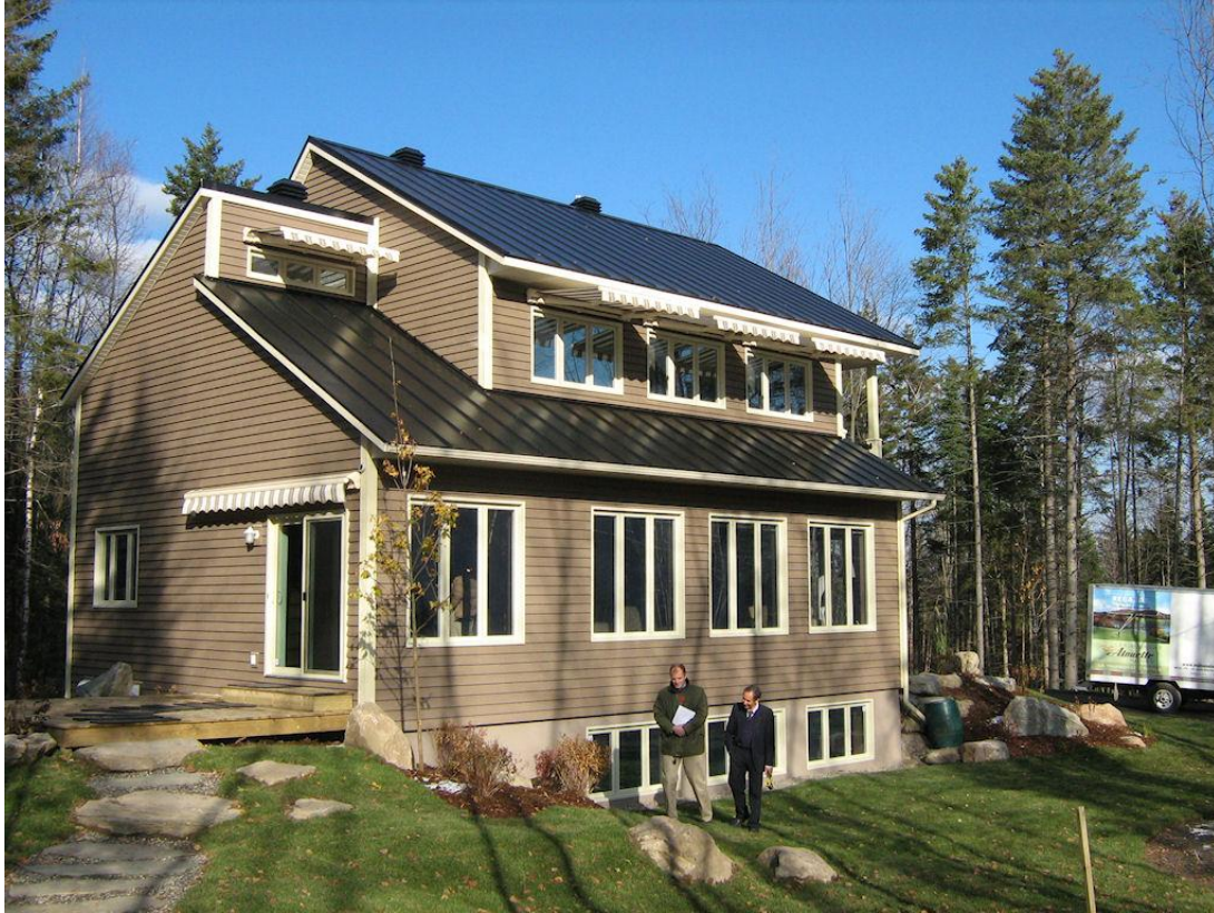
Figure 2-18. Alouette Ecoterra EQuilibrium House with BIPV-T Roof The photovoltaic panels are integrated with the architecture of the house Source: www.cmhc.ca
