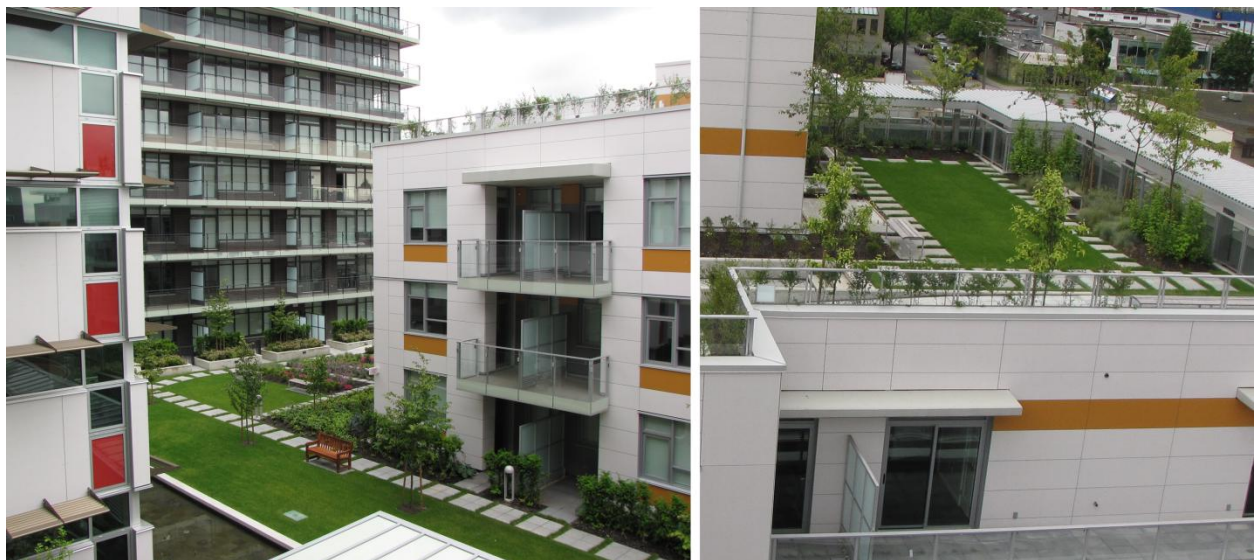
Figure 4-1. Green Roofs Widely Used in Buildings in the Olympic Village. Green roofs can be used to enhance the architectural quality of the space as well as to help the building to avoid sun's heat.
