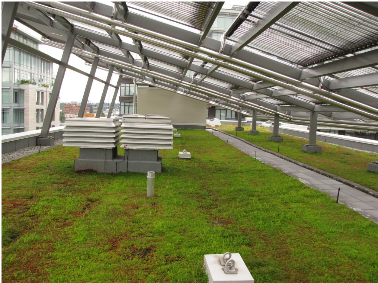
Figure 3-56. Evacuated Solar Tubes on a steel structure The picture shows how the architect has used both evacuated tubes and green roof in his design
