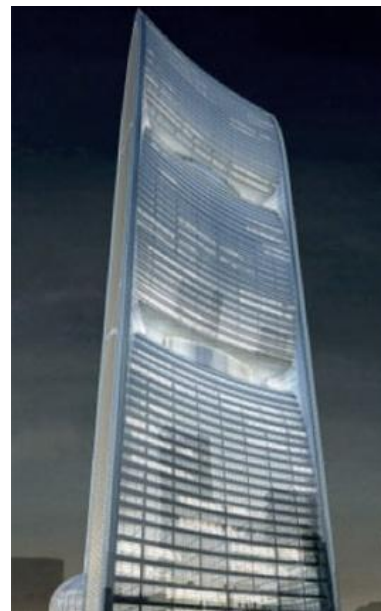
Figure 2-29. Pearl River Tower, China - The design contributes to the wind turbines to produce energy Source: www.sustainabledesignupdate.com - www.greendiary.com
