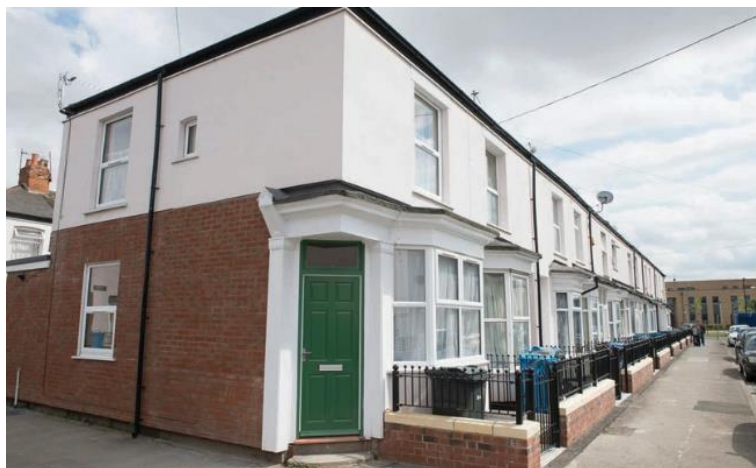
Figure 2.1: Giroscope housing after reconstruction
