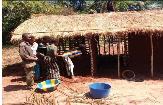
Figure 3.5: Construction process of a shelter by the refugees
