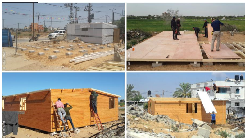
Figure 3.41: Construction Process of the shelters
