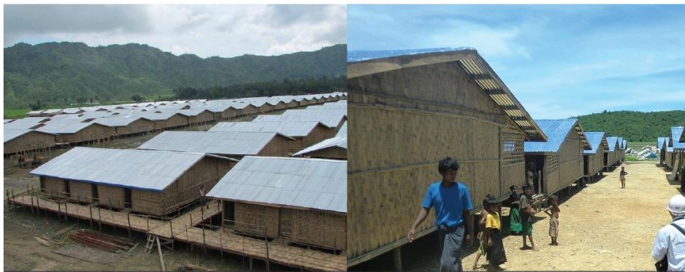
Figure 3.13: Elevated shelters for the IDPs after completion
