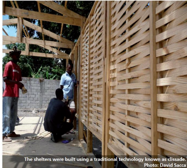
Figure 3.36: Shelters built using traditional clissade technology.
