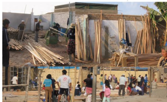
Figure 3.32: Construction process of the prefabricated shelters
