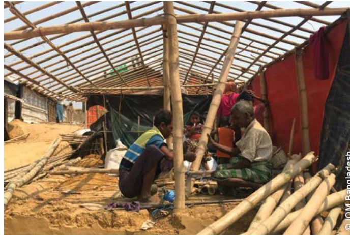
Figure 2.12: Self-help shelter construction process by the refugees.
