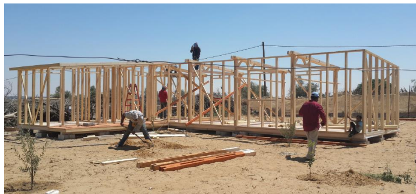
Figure 3.42: Experienced workers built the structure as timber construction was new in the country
