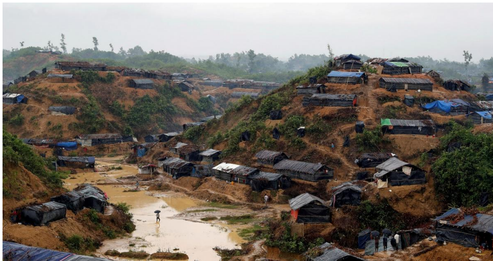
Figure 2.6: Condition of Rohingya camps during the monsoon.
