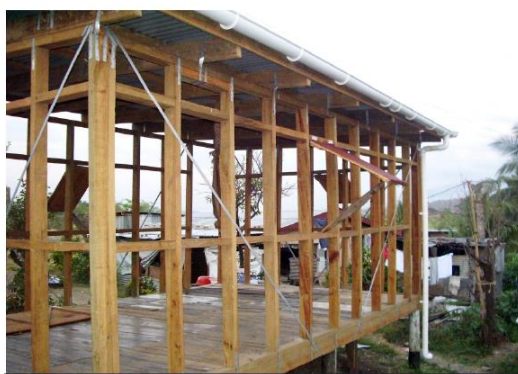
Figure 3.46: Construction process during a prefabricated shelter
