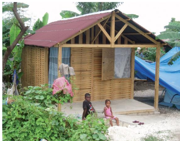
Figure 3.34: A completed prefabricated shelter assembled by the beneficiaries
