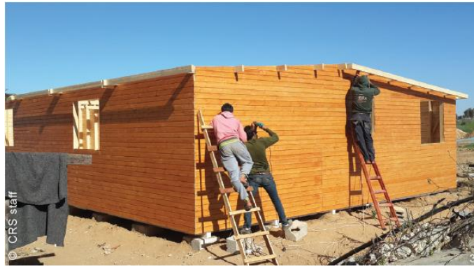
Figure 4.3: A prefabricated refugee shelter in Gaza assembled by the beneficiaries themselves.
