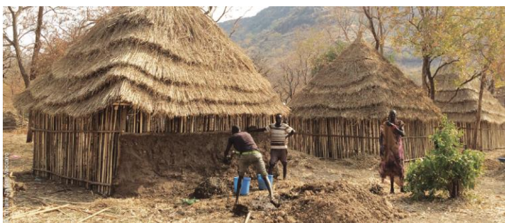
Figure 3.18: Construction of tukul houses by the beneficiaries.
