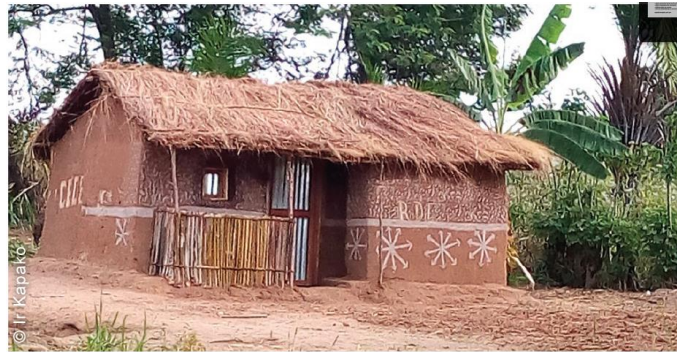
Figure 3.1: Shelters built by the communities
