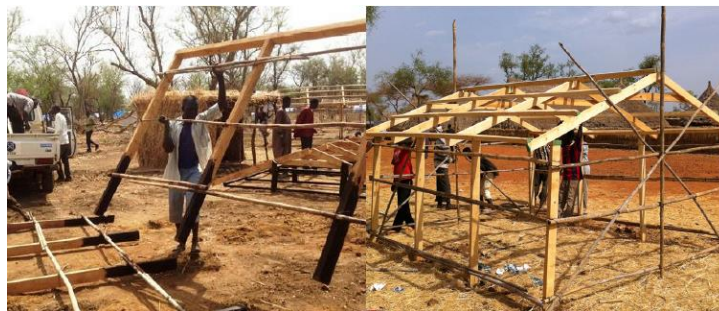
Figure 3.24: Construction of the shelters by the beneficiaries
