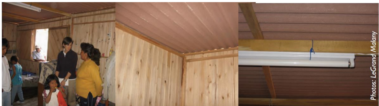
Figure 3.30: Prefabricated shelter built on the roof of a destroyed house
