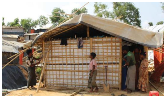
Figure 2.18: Upgraded shelter made of bamboo structure and tarpaulin.
