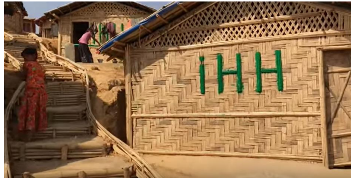
Figure 4.6: A bamboo shelter in Rohingya refugee camp in Bangladesh
