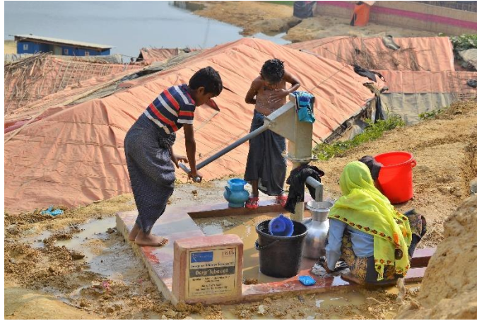
Figure 2.7: Deep tube wells in the refugee camp for drinkable water
