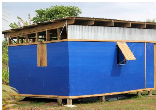
Figure 3.44: After construction of the prefabricated shelters by the beneficiaries.
