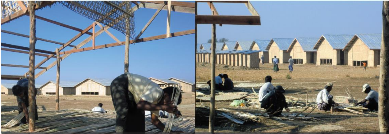
Figure 3.15: Shelter construction by the IDPs
