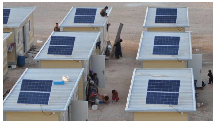
Figure 4.9: Solar panel on refugee shelters in a refugee camp in Syria.
