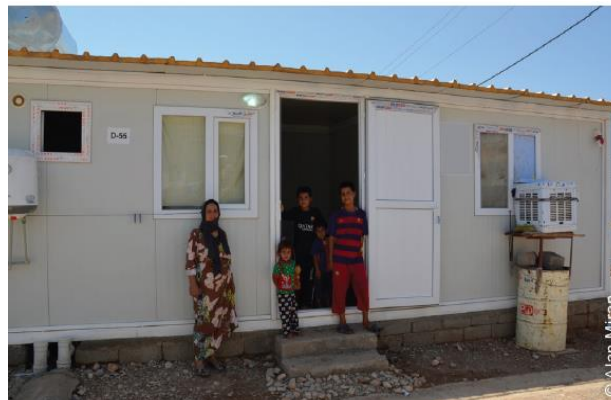
Figure 4.5: A prefabricated wood shelter for refugees in Iraq.
