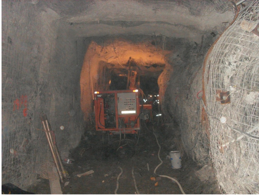
Figure 4.7 Footwall closure at Lapa mine.
