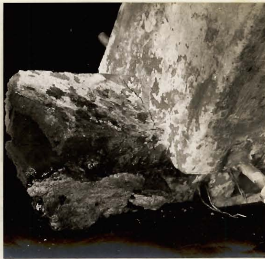
Fig. 43. Inlet failure, Bacite removed
