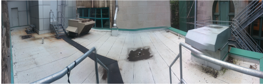
(a) McGill McDonald Engineering Building Rooftop Picture
