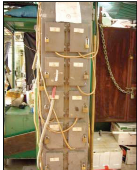
Figure 5.5: Electrical outlets behind Temple Street Market stalls (Source: Zunn, 2006)
