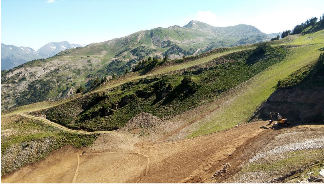
Figure 43. Visual aspect of the ski run down from the north face curve during the works to reshape the mountain slope (15/7/2018).
