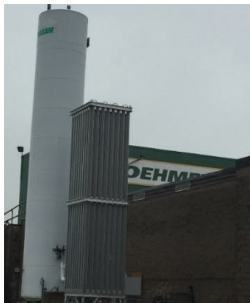
Figure 3.14: Pure CO 2 pressure tank for the early carbonated curing process
