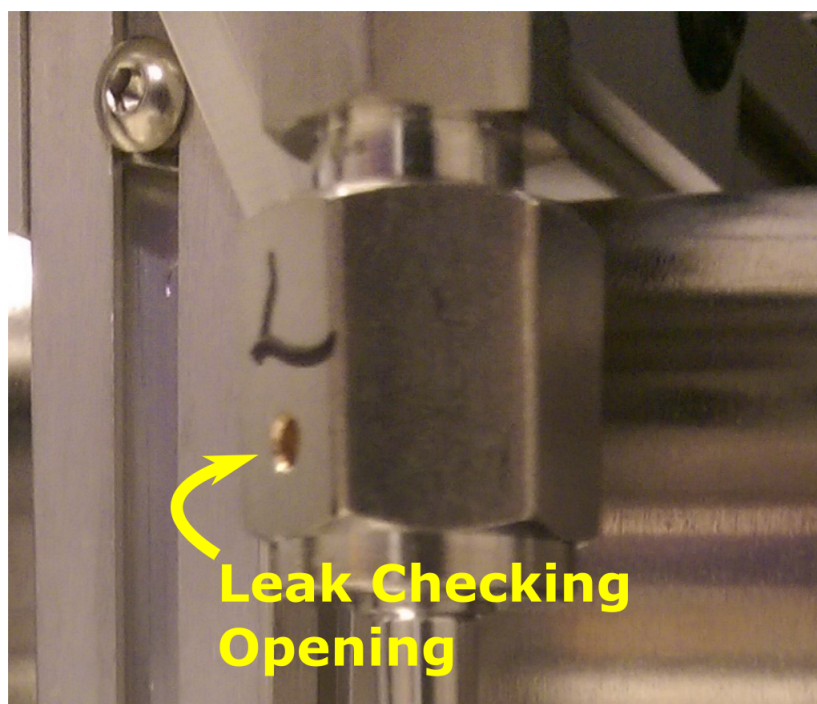
Figure 24: Male-female VCR junction with leak checking hole. When leak checking, He gas or ethanol is sprayed into every single junction whose gasket has been changed.
