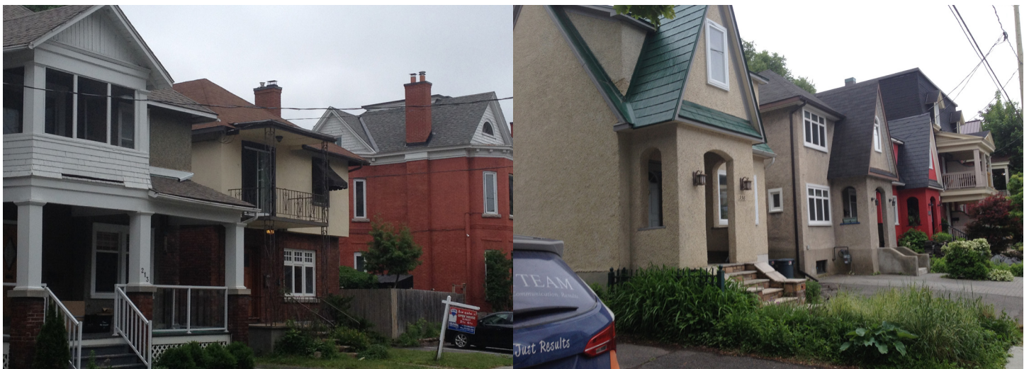
Figure 11: (Left and Right)) Examples of traditional building materials of stucco, brick and wood siding that have been conserved, 2016, however some elements like the front railings and historic metal roofing have been lost.
