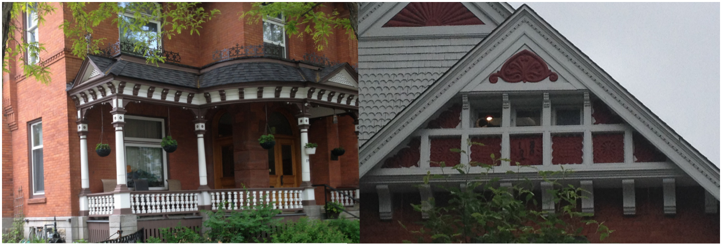
Figure 9: (Left) Painted wood front porch with prominent brackets , 2016 and (Right) Intricate trim work set into the gable , 2016; elements that have been conserved over time.
