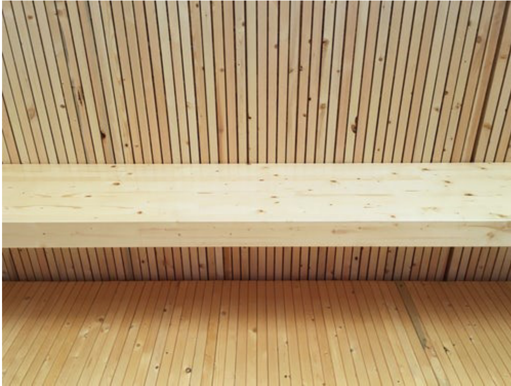
Figure 23 - Ceiling made of nail-laminated timber. (N. R. Canada 2014)
