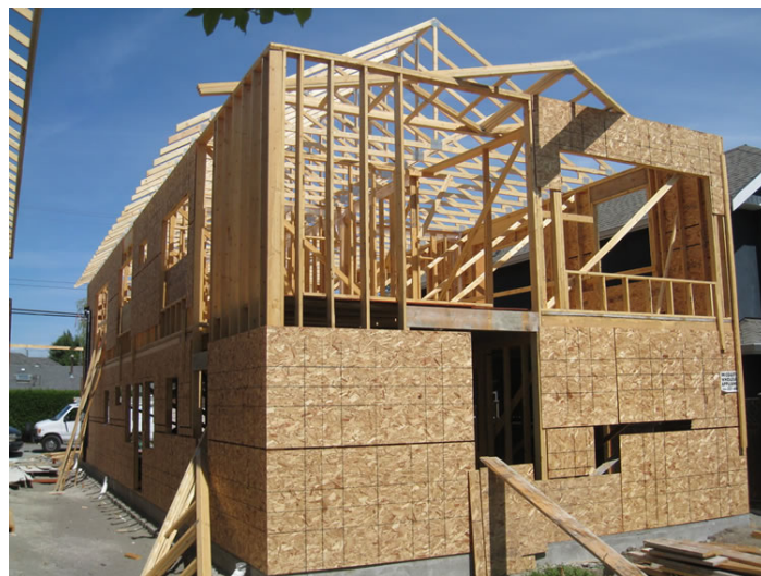
Figure 20 - OSB used as sheathing in residential construction. (Photo: N. R. Canada 2014)
