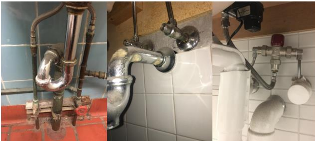
Figure 3.1 Visual inspection a) copper, b) maybe, c) not identifiable
