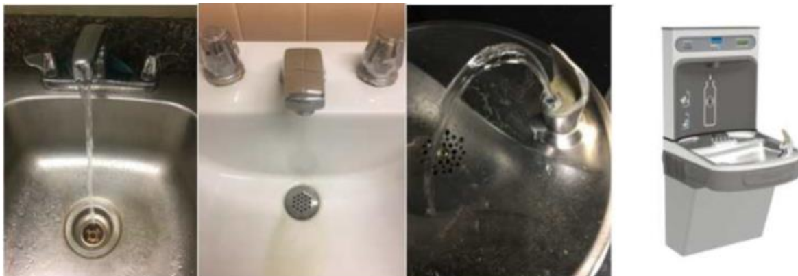
Figure 3.2 Examples of water outlets from which water samples were collected. a) water fountain with filter, b) regular water fountain, c) newer sink, d) older sink
