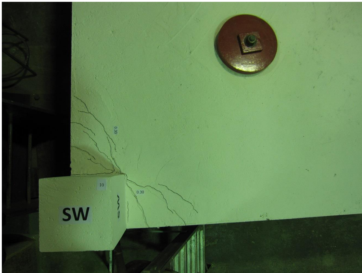
Figure 3-36: Crack pattern around corner slab-column connection SW at load stage 10
