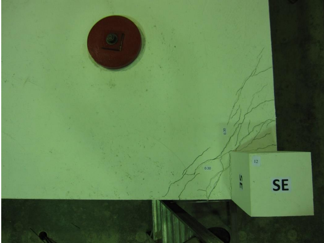
Figure 3-52: Crack pattern around corner slab-column connection SE at load stage 12
