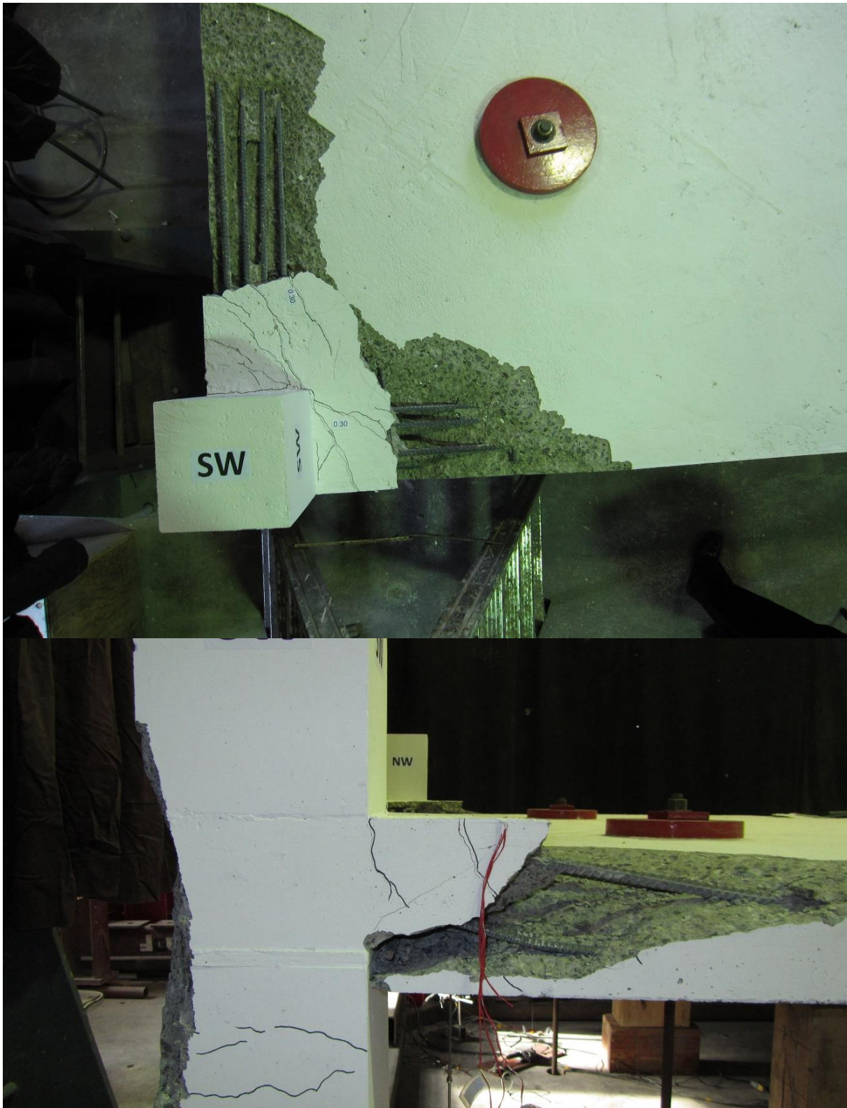
Figure 3-35: Post-punching shear condition of the corner slab-column connection SW at the end of testing
