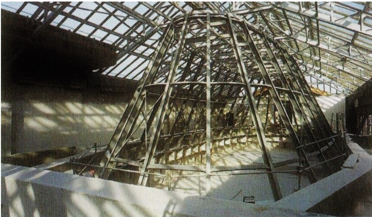
Figure 61. Skeletal support of conic structure built atop the rooms of the Orangerie Water Lilies gallery, 2000-06. Musée de l'Orangerie, Paris. Photograph by © Agence Brochet/Lajus/Pueyo in Pierre Georgel, Le Musée de l'Orangerie (Paris: Gallimard – Réunion des musées nationaux, 2006), [n.p.].
