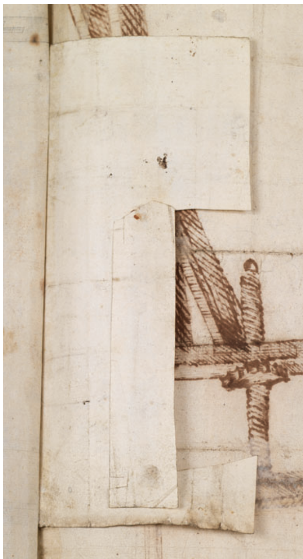
5 Verso of Robert Hooke's drawing of Towneley's micrometer revealing where and how it has been cut and pasted back together, autumn 1667. 90 × 199 mm. London: Royal Society (Classified Papers, 2, 13). Photo: © The Royal Society.
