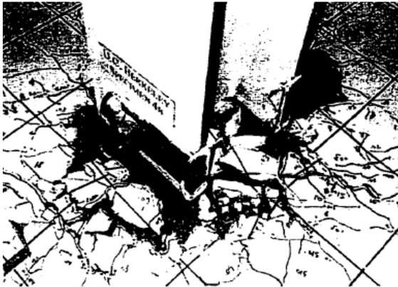
(c) crushing of concrete slab
