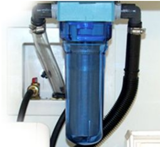
Figure B1: Lint LUV-R filter after installation (credit: http://www.environmentalenhancements.com )
