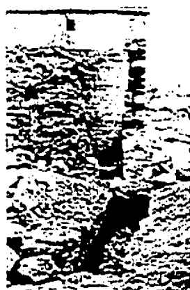
Upgrading a wall after demolition - from cob to composite masonry at Lidhora
