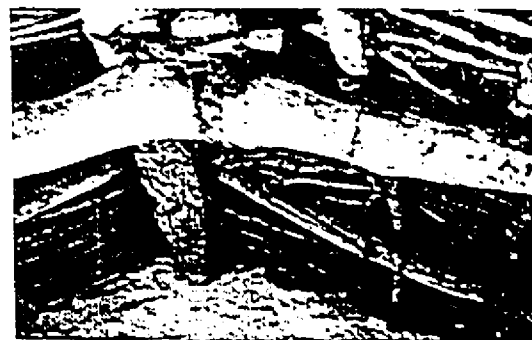
Under-structure of a khaprel roof
