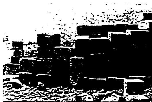
Hand-tamped concrete blocks, Pura Badhera
