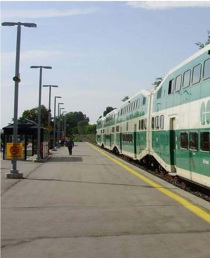
GO Train Platform, Toronto, TRAM
