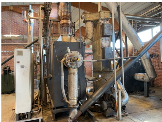
Figure 5: Bio-oil combustion connected to a local district energy system (DES) in Hiedanranta, Tampere, Finland. Author photo.
