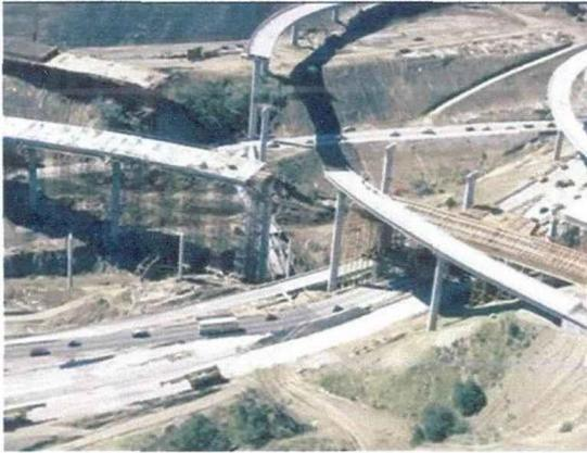
**Fig 1.1 Failure of the SR14/15 Interchange**
