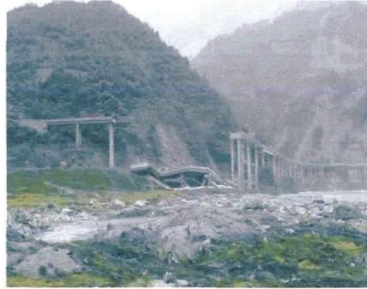
**Fig 1.2 Failure of the Baihua bridge**
